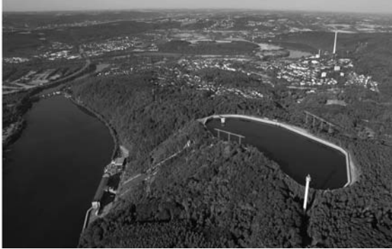
Figure 4.16 Koepchenwerk pumped-storage facility with a net storage of 1.5 million m 3 located along the Hengsteysee reservoir on the Ruhr River, near Dortmund, Germany.
