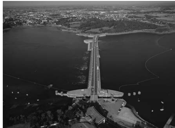
Figure 4.12 The Rance Tidal Power Station produces electricity with 24 turbines and has a peak electrical power output of 240 MW.
