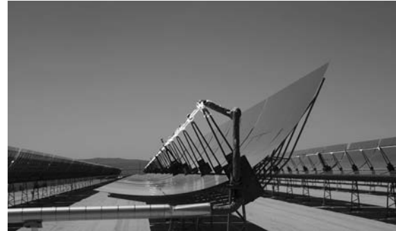
Figure 4.8 Parabolic mirror arrays of Solar Energy Generating Systems (SEGS) facility in the U.S. Mojave Desert.
