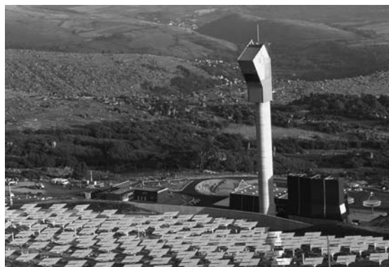
Figure 4.5 THEMIS Solar Tower Power plant near Targassonne in the Pyrénées-Orientales of France.
