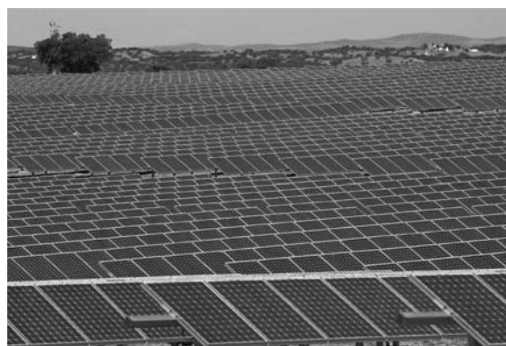
Figure 4.10 Photovoltaic power plant at Serpa, Portugal that includes a tracking system to follow the sun’s path across the sky.
