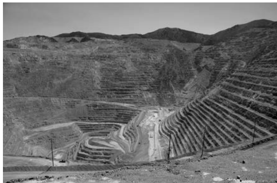
Figure 1.3 Bingham Canyon copper mine in Utah is the largest excavation (Over 4 km wide) and the deepest open pit mine (Over 1.2 km deep) in the world.
