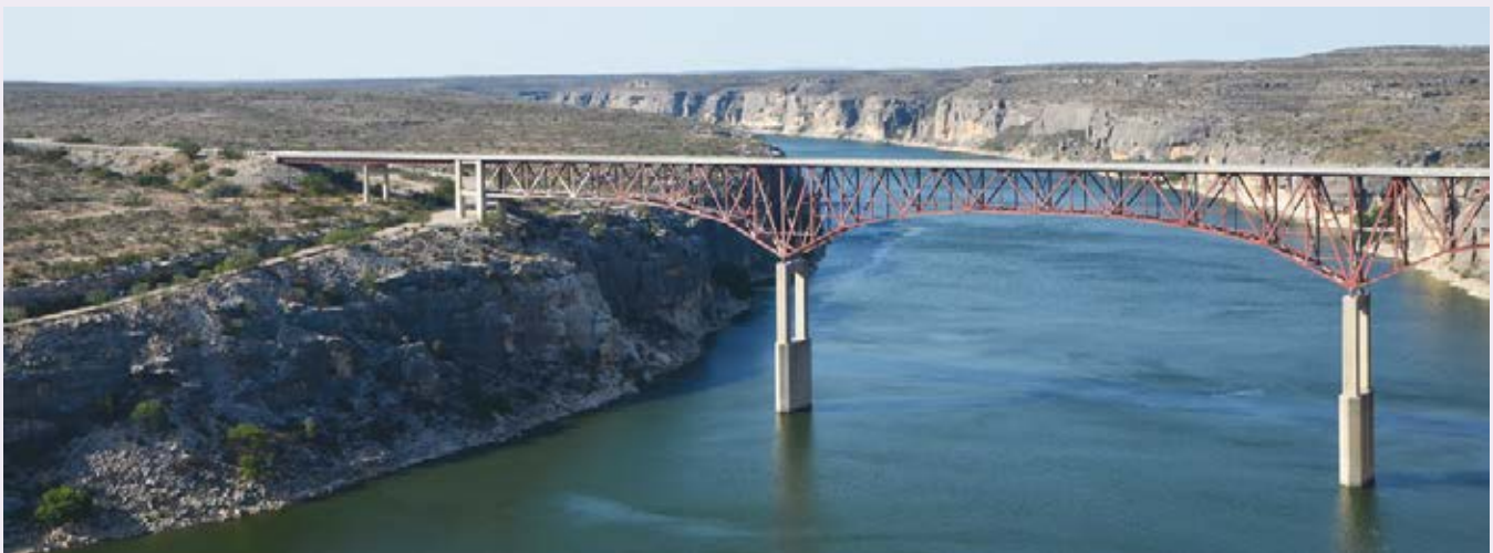
FIGURE B1-3 Limestone is calcium carbonate, composed of the shells of sea animals such as clams, mollusks, and certain algae. As these creatures formed their shells, they removed carbon dioxide from the atmosphere, causing the climate to become cooler. All the rock in this area along the Pecos River is part of a gigantic region of limestone that extends for hundreds of square miles.
