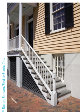
Stairs showing a stringer
