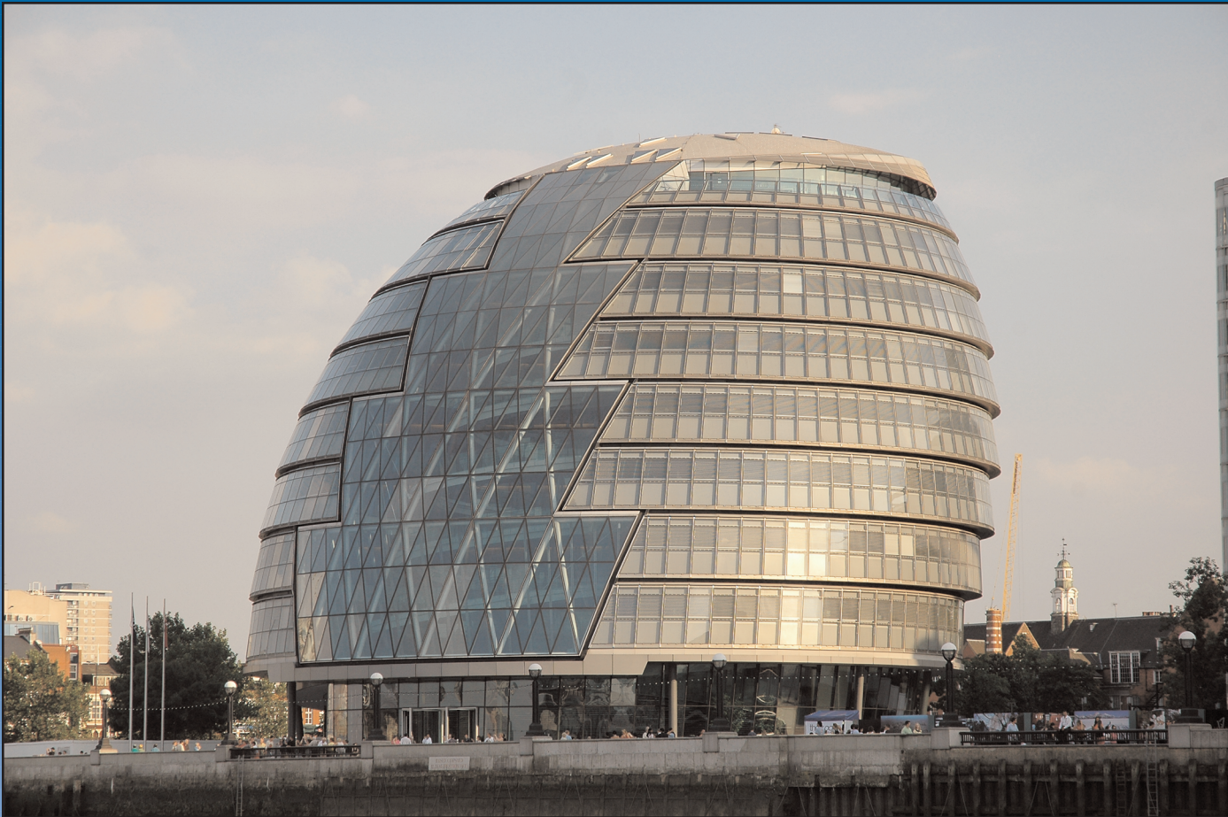
City Hall in London, England, stands on the left side of the River Thames, in the More London development by Tower Bridge. The building, designed by British architect Norman Foster, was opened in 2002. Its bulbous shape reduces surface area and thus improves its energy efficiency.
