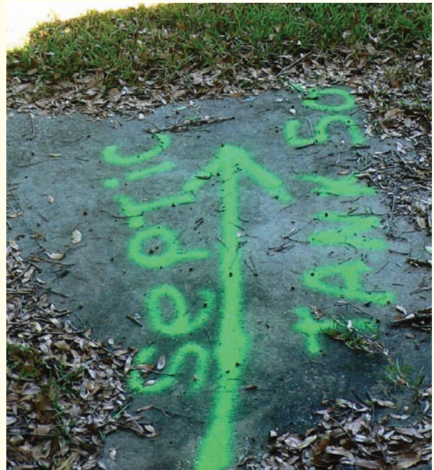
Figure 6-1 Septic tanks and other hazards should be marked for safety.
