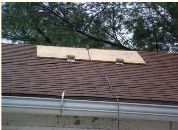
Figure 6-7 Roof ventilation openings are made during preparation, not during the actual fire. Hinges, pivot, and cable allow remote release from the ground.
