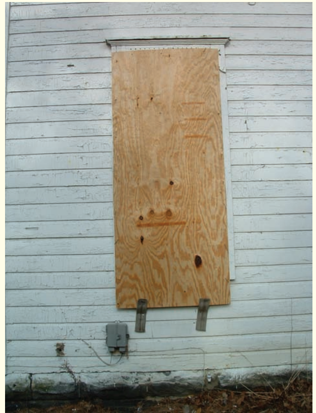
Figure 6-3 Hose hinges keep window coverings in place, but are easily knocked down.
