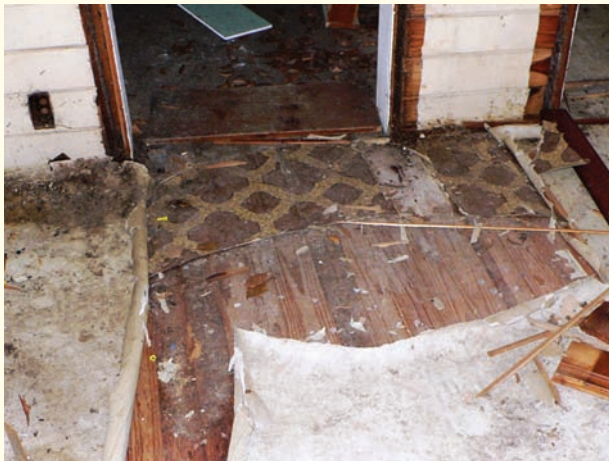
Figure 6-8 For safety, expose the structure's actual floor by removing all additional layers of flooring.
