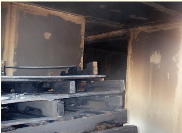
Figure 6-13 Greater fire resistance can be added by lining the burn room with drywall.
