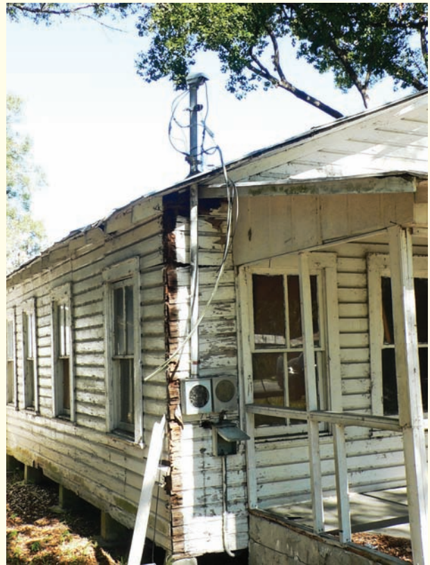
Figure 6-5 Ensure that the electrical service lines are disconnected from the pole to the weather head.
