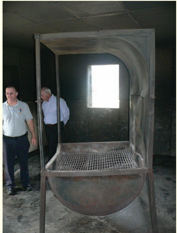
Figure 6-14 Hearths or fireboxes can protect the ceiling to allow for more live fire evolutions.
