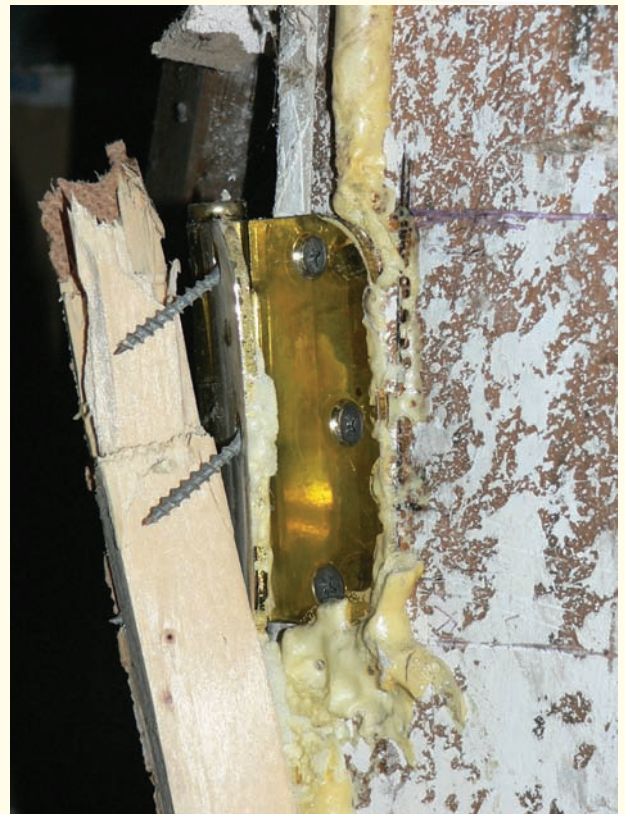
Figure 6-9 Any hardware that may snag or catch on PPE must be removed.
