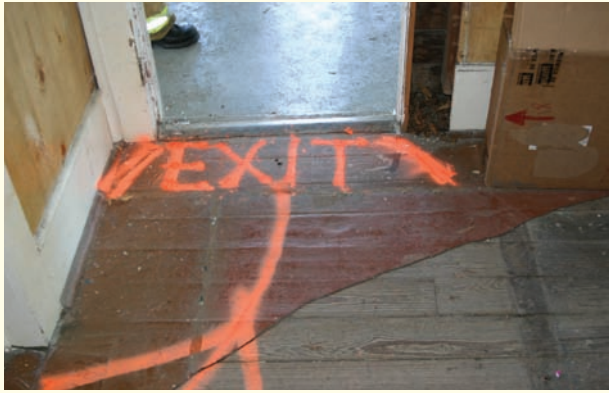
Figure 6-12 Fluorescent spray paint can be used to mark the way out.
