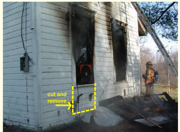
Figure 6-4 A window can be made into a doorway by cutting and removing a section of the wall below the window.
