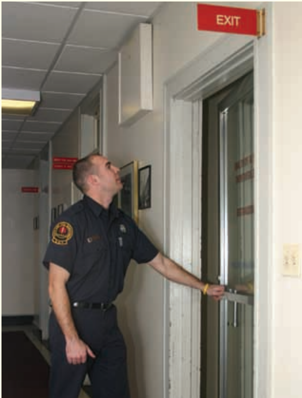
Figure 16 Means of egress must be inspected.
