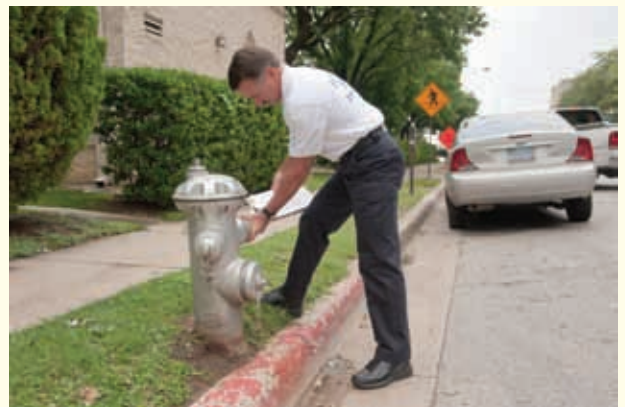
Figure 10 From the exterior you can observe vehicle access, fire lanes, fire hydrant access, or caps missing on fire hydrants.
