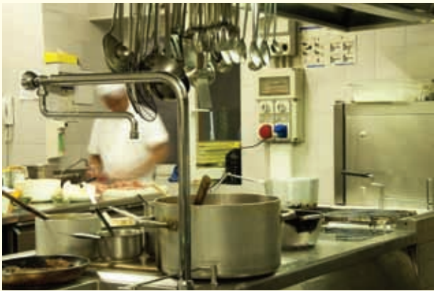
Figure 12 A kitchen may call for a specialized fire suppression system.
