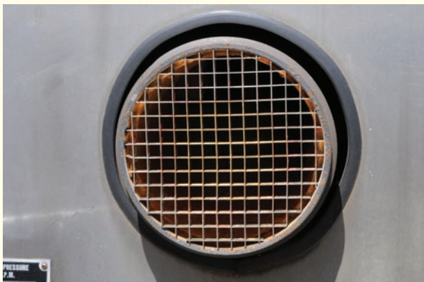
Figure 6-21 The strainer should be in good condition and should not have any missing or damaged pieces.
